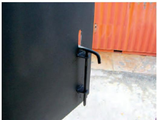
**Figure C-6: Window & Latch Construction**
